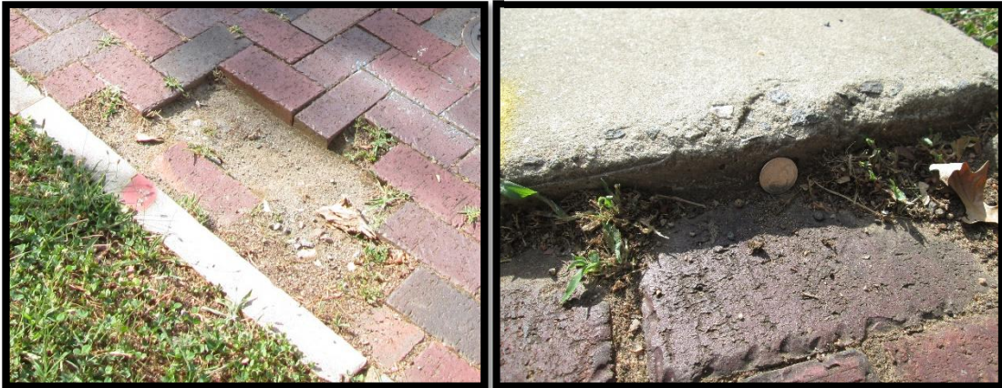
Figure 20 and Figure 21: Tripping Hazards on Catawba Avenue Sidewalks (Typical)
