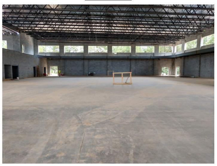
Area C-Gym roof joist & deck installed. Track steel being installed.
