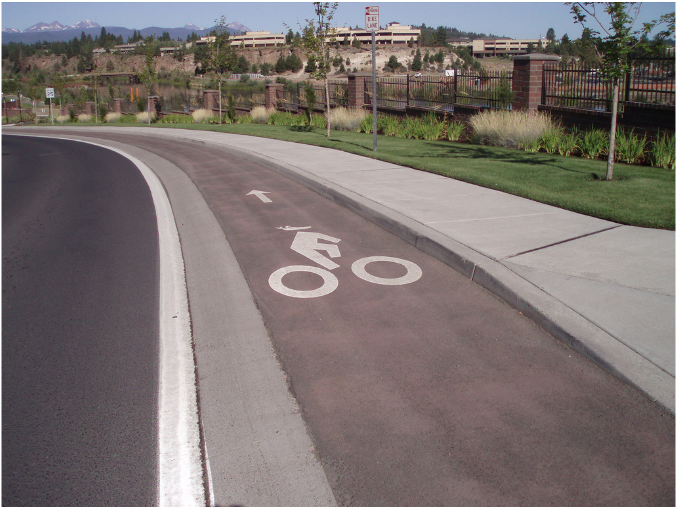
Raised Cycle Track: Bend, OR.
